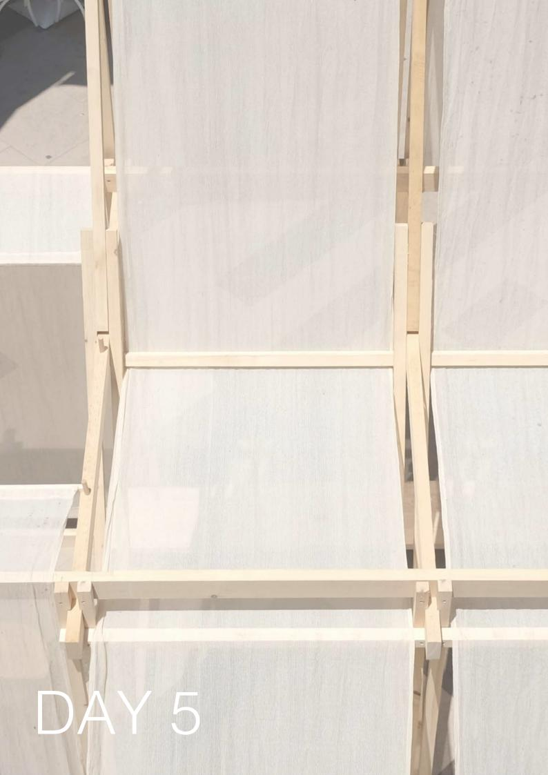
With the collaboration of the fashion department, the **agriculture mesh** was dimensioned in length, reinforced on the sides and pockets where added to its extremes to hold sticks that where to be sustained with cords, and then attached to cellular concrete blocks for tension.
